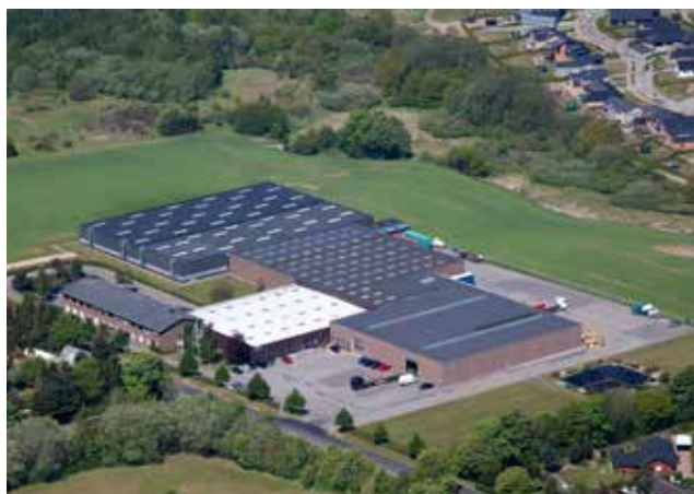
ERMAX A/S, Kolding, Denmark
